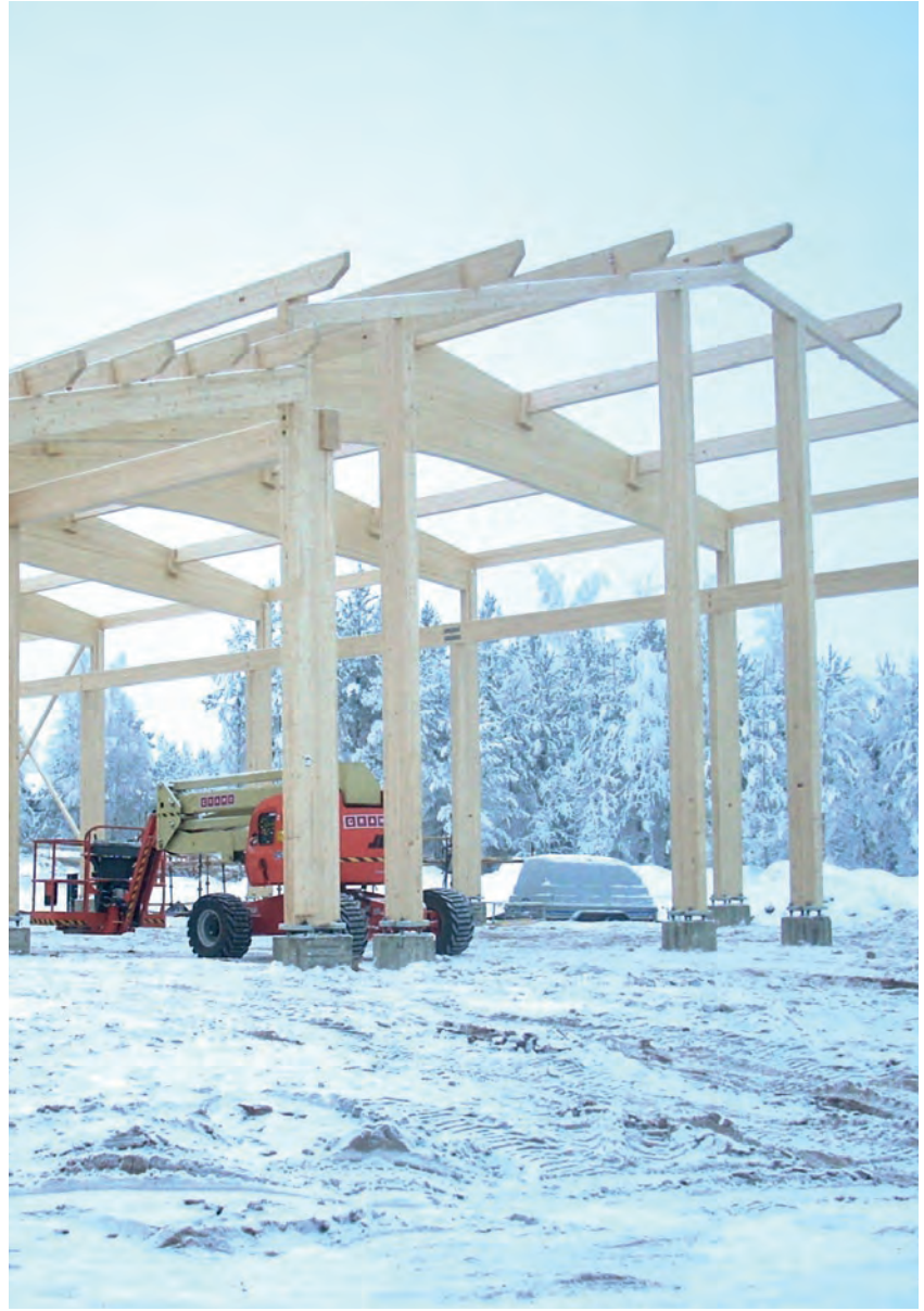
Industrial Hall, Valkeala
