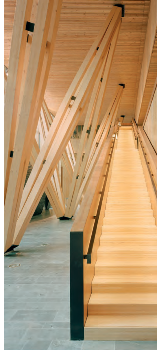
The Metla Building, The Finnish Forest Research Institute Joensuu
